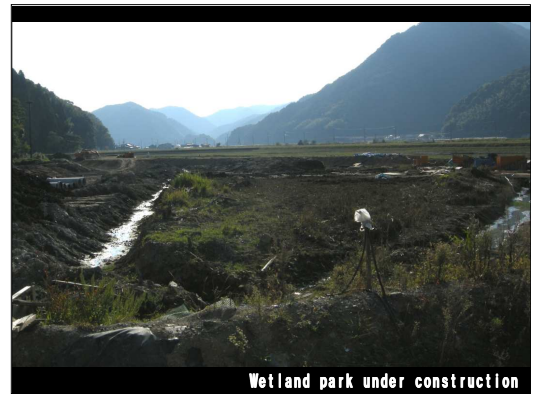
Wetland park under construction
