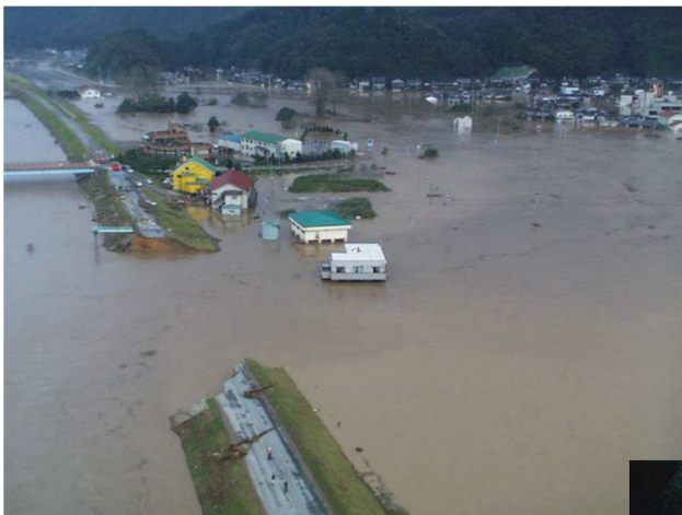
Flood damage caused by Typhoon no.23 in 2004.
